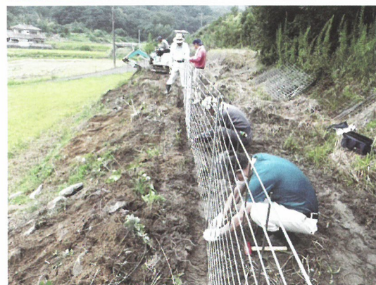
侵入防止柵の点検・補修
