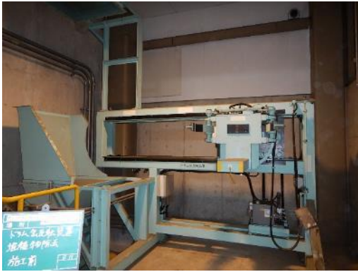
除去・除染作業前
