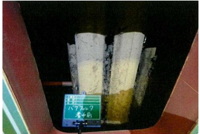
除去・除染作業前
