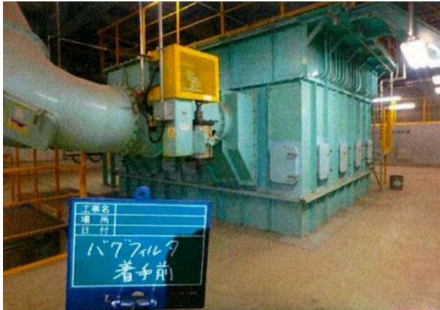
除去・除染作業前
