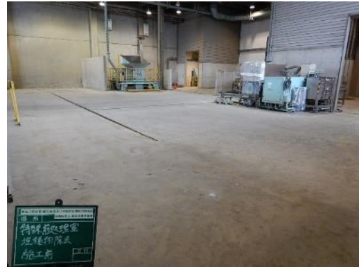
除去・除染作業前
