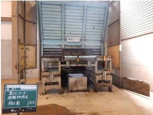
除去・除染作業前
