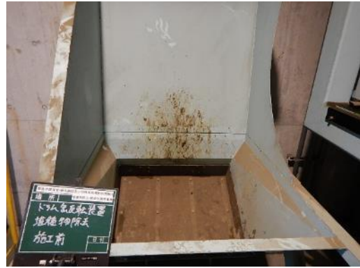
除去・除染作業前
