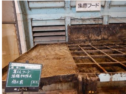
除去・除染作業前
