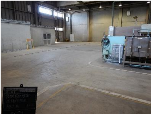
除去・除染作業前
